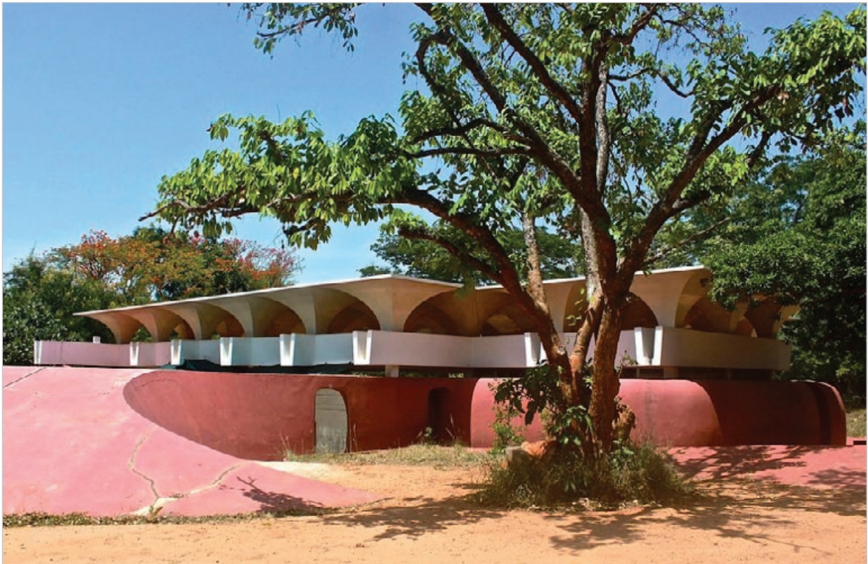
Original Last School building
