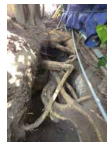
Figure 2 Trench to install utility line excavated by pneumatic excavator
