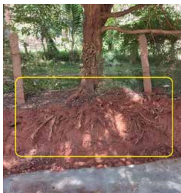
Figure 2 Trench to install utility line excavated by pneumatic excavator
