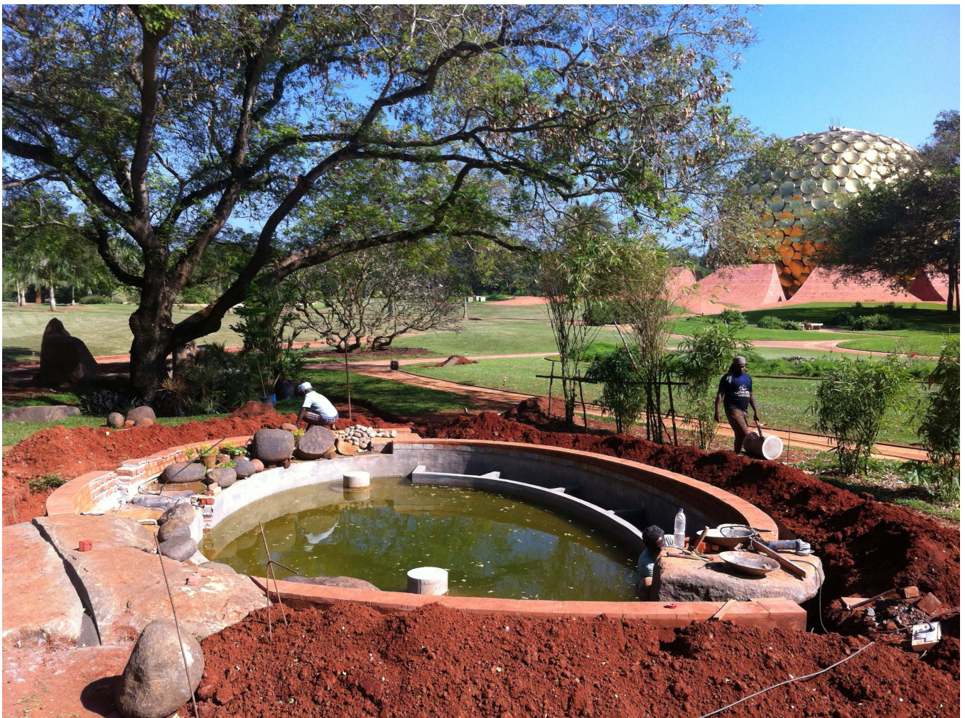
Building the new pond in the Garden of the Unexpected
