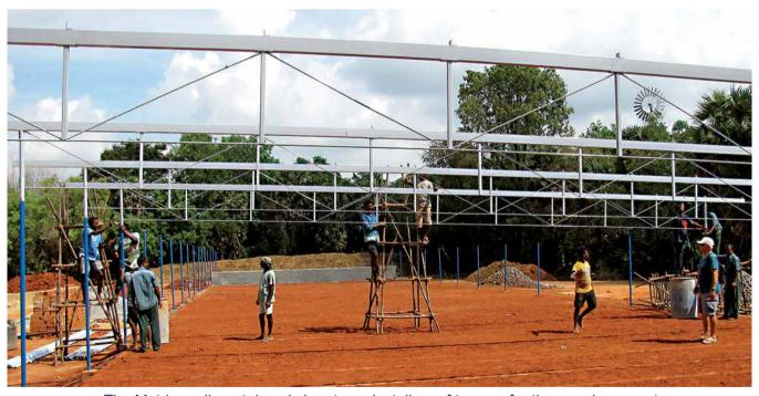
The Matrimandir metal workshop team installs roof trusses for the vermi compost production shed at the new site.
