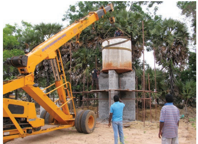
Work takes a step forward at the new location for compost production for the Matrimandir gardens, with the installation of an overhead water tank on June 30th. The next step will be the construction of a shed for vermi-compost production.
