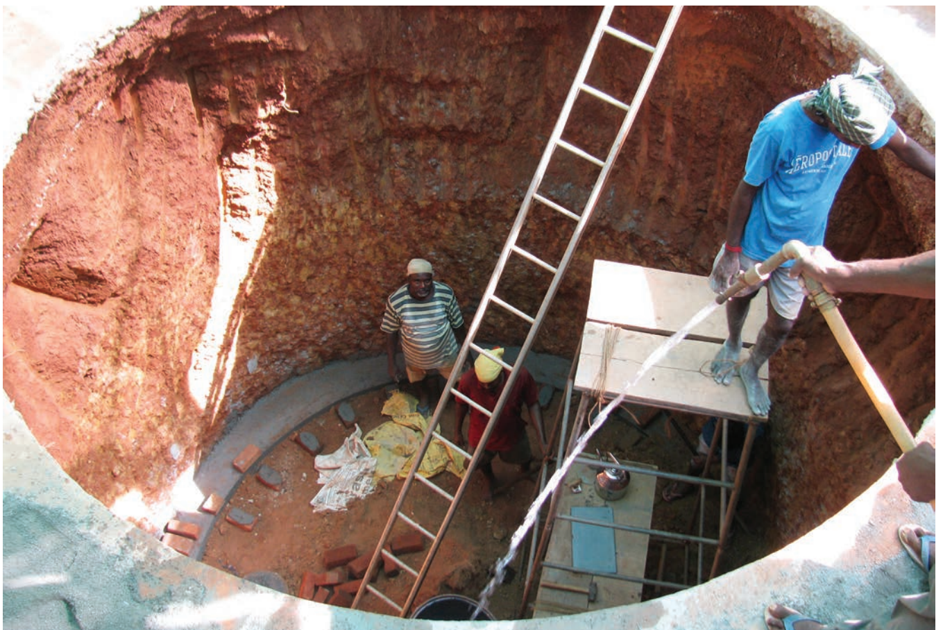
Masons begin to build the brick walls of the deep open well which will receive runoff rain water from the Amphitheater. Pumps located here will then send the harvested rainwater into the open water channel being now constructed around the gardens oval.
