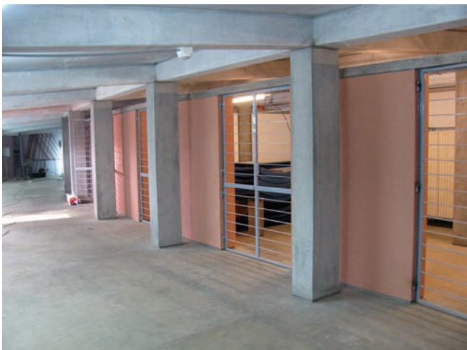
The Garden Tools Center beneath the Western rim of the Amphitheater has been under construction for the last two years and is nearly complete. This space will be the center for storage and distribution of garden tools for the maintenance of the Matrimandir gardens over the generations to come.
