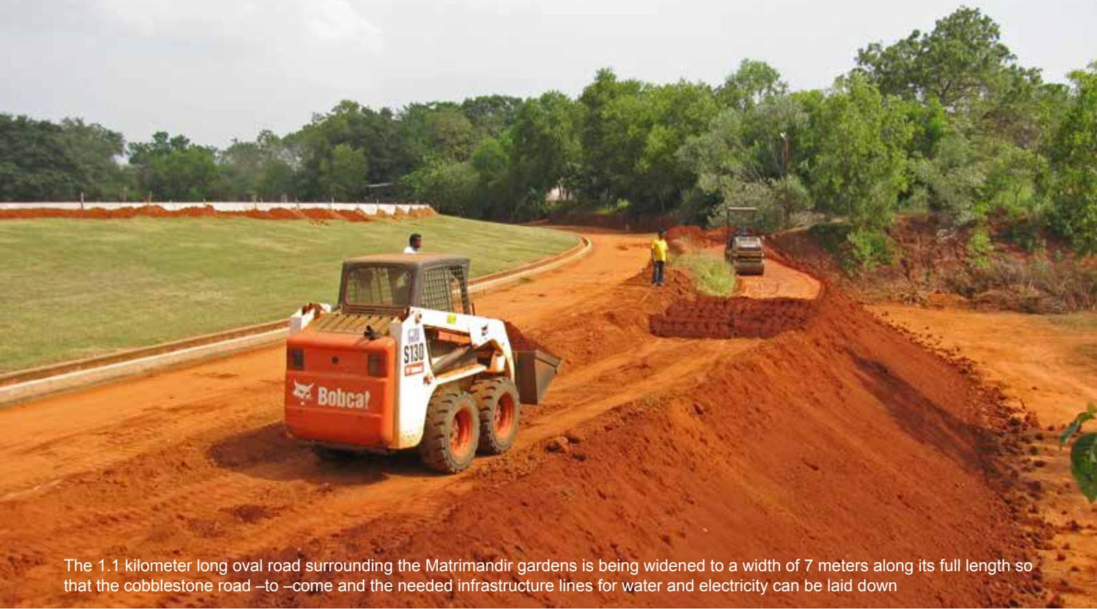
The 1.1 kilometer long oval road surrounding the Matrimandir gardens is being widened to a width of 7 meters along its full length so that the cobblestone road –to –come and the needed infrastructure lines for water and electricity can be laid down
