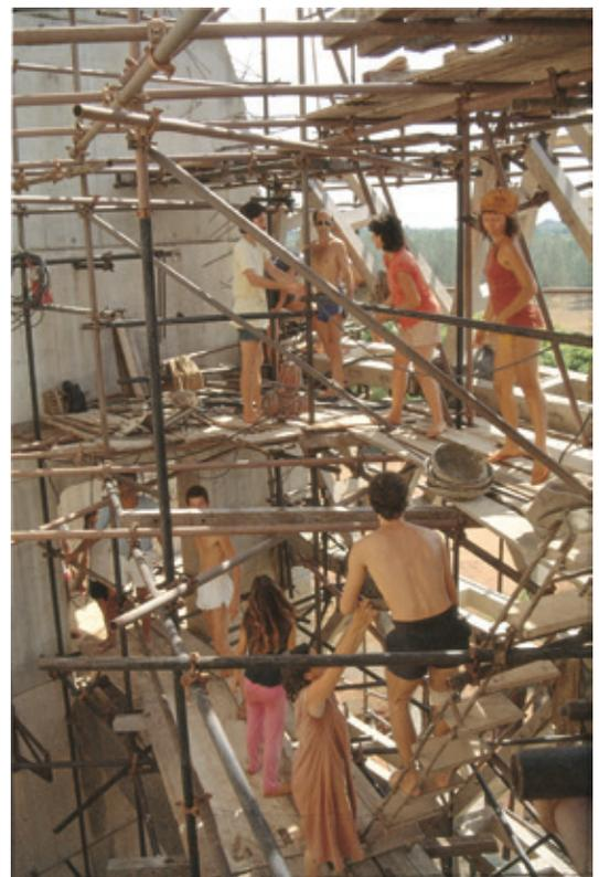
A human chain lifts chetties of concrete up to fix a new row of the space frame beams in place.
