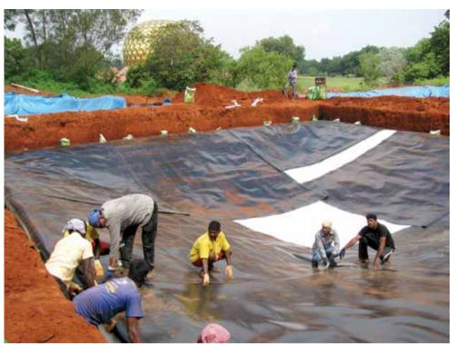
from its surface. Another Construction. The joints of the HDPE were welded together by a marvelous self propelled type of sealant, made of robot welder which formed a perfect double seam. The seams were then subjected to strict a Plastic foil, (HDPE) two mechanical tests to ensure that there were no leaks in the sealant layer.
