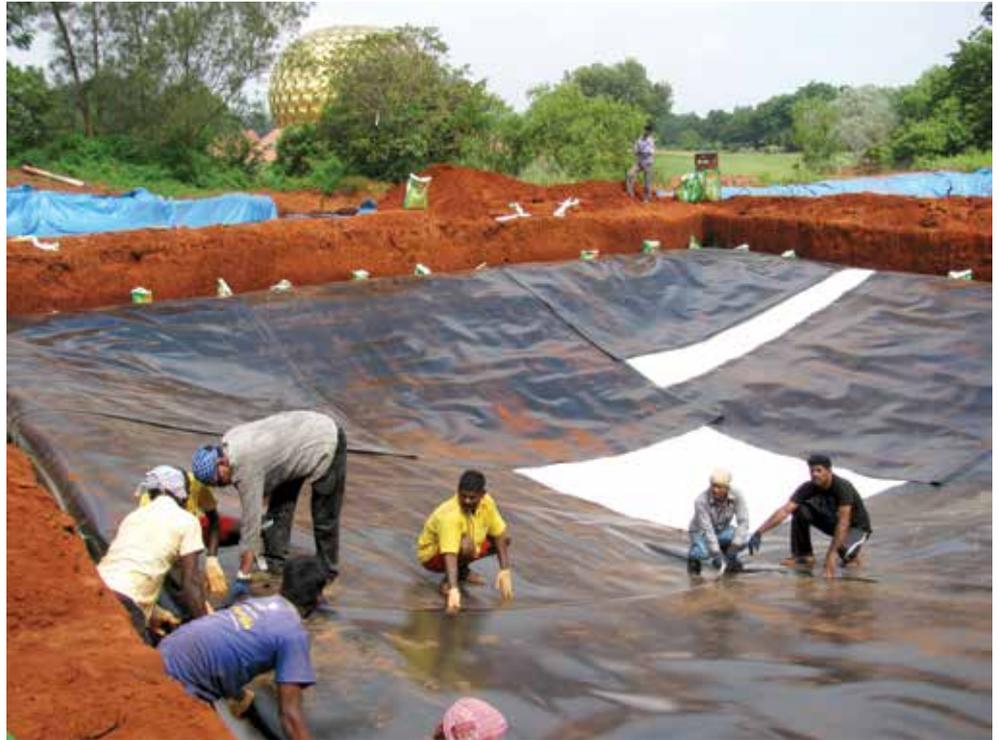
One of the two mini test ponds which are sealed with HDPE foil is shown here under construction. The joints of the HDPE were welded together by a marvelous self propelled robot welder which formed a perfect double seam. The seams were then subjected to strict mechanical tests to ensure that there were no leaks in the sealant layer.
