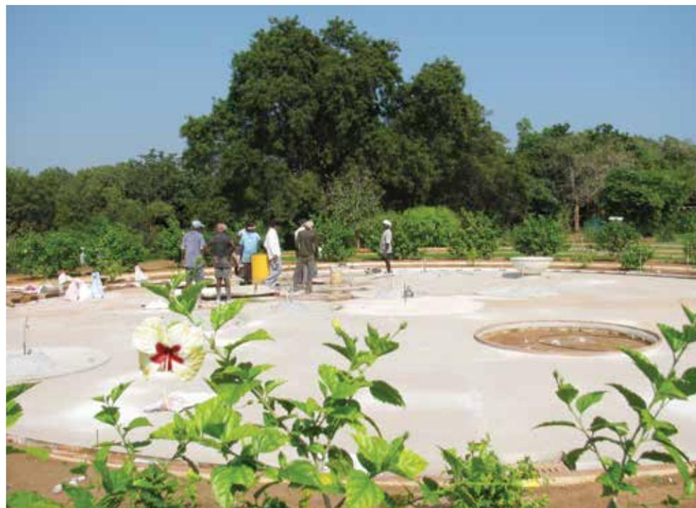
A wide level base of lime and pebbles is laid down in the center of the garden of Bliss in mid January. Once the seven bowl-shaped fountains are in place, this circular area will be finished with a layer of loose, white quartz pebbles.
