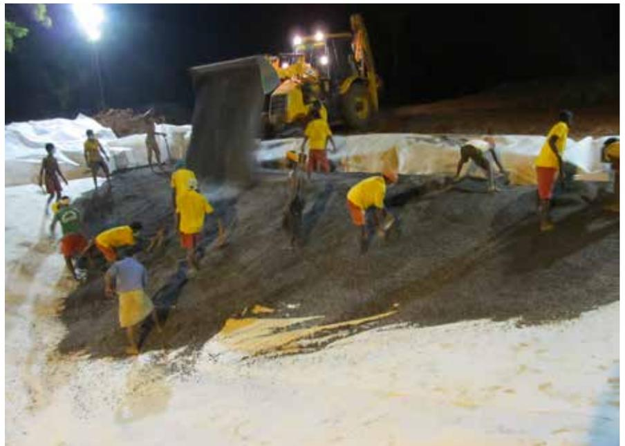
The sealed clay layer was covered with a protective layer of white geotextile, and then with a thick layer of granite chips.
