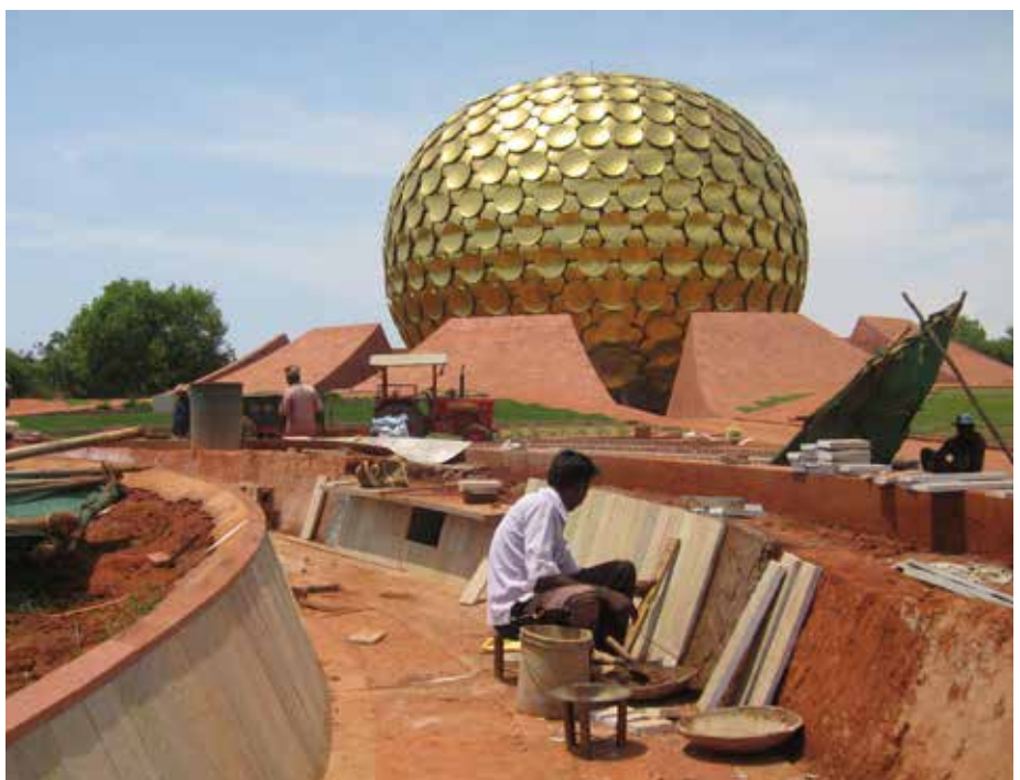
Slate stones are fixed against a backing of lime and red earth mortar to create the "sunken path" in the Bliss garden.
