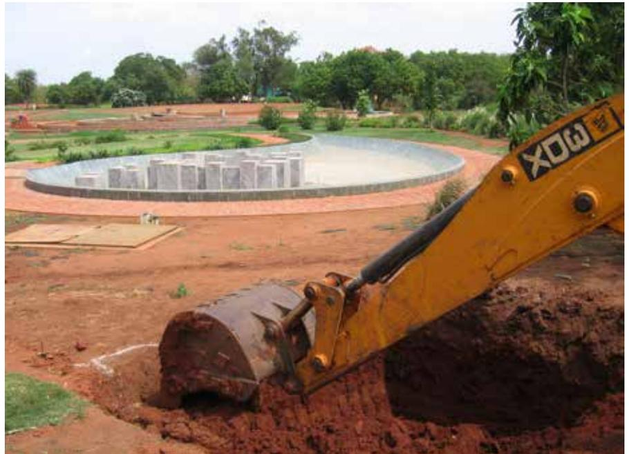
A JCB started on June 25<sup>th</sup> to dig the hole for the underground pump room in the Garden of Consciousness
