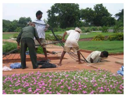
Electric cables powering pumps and lights in the first three gardens are rerouted under the pathways to go to the new underground control room in the Garden of Consciousness.
