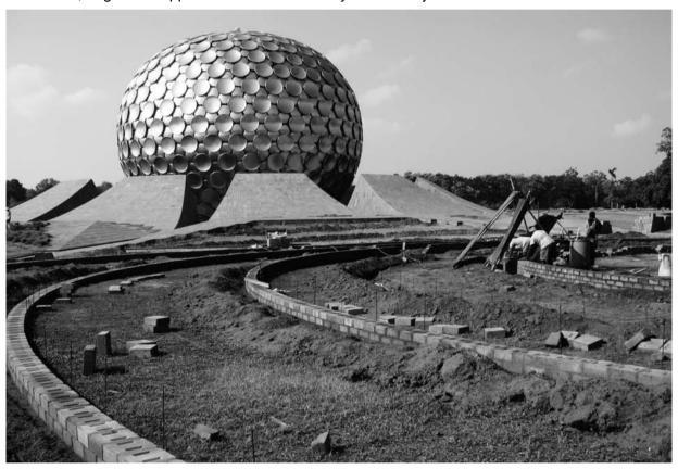
Building the compressed earth block walls in the garden of Bliss
