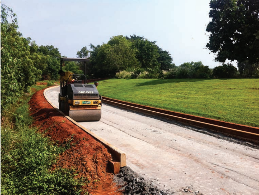
A portion of the oval road, 130 meters long is being prepared for its surface cladding of granite cobble stones.
