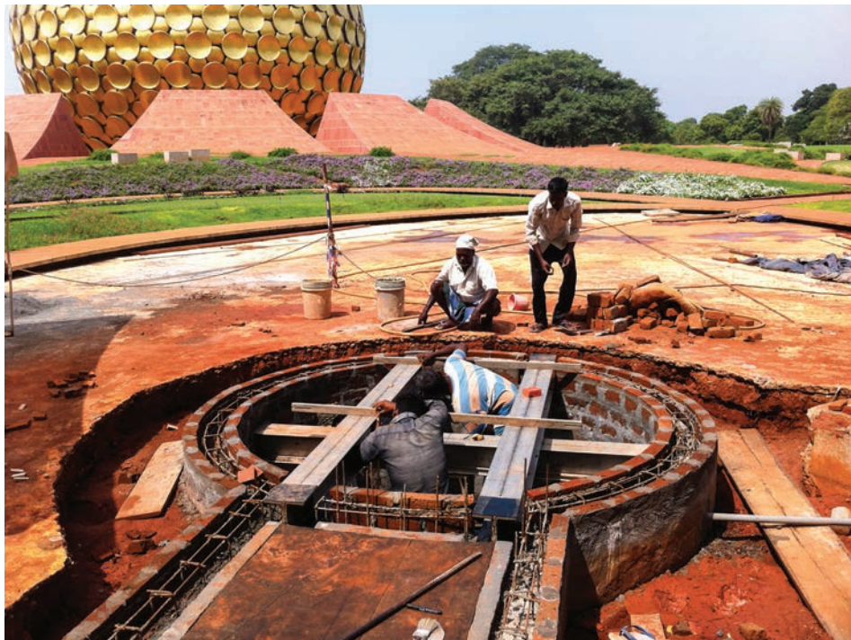
The concrete foundation for the crystal group in the garden of Existence being completed in October.
