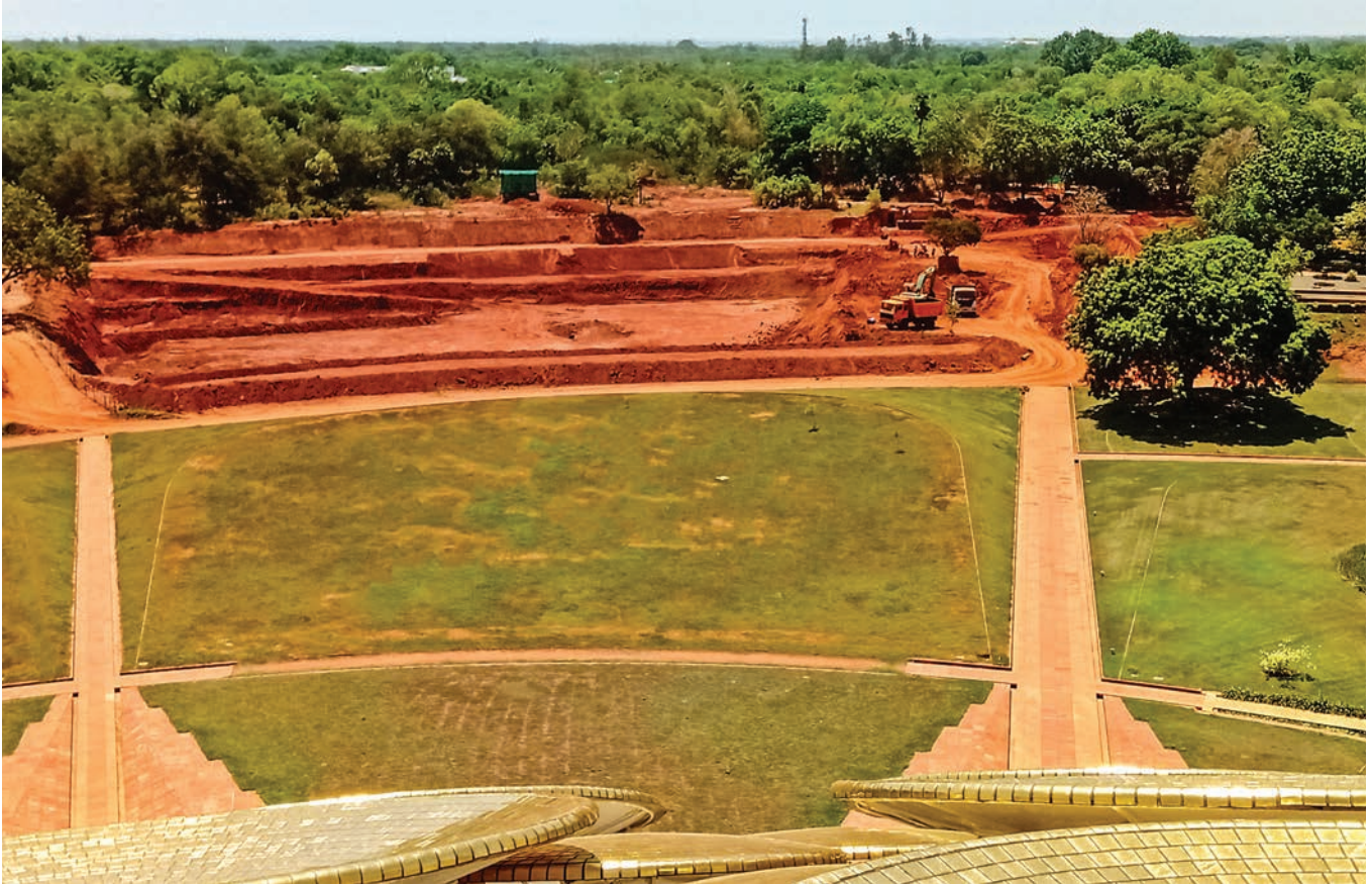
The Test Pond excavation as seen from the top of Matrimandir during September.
