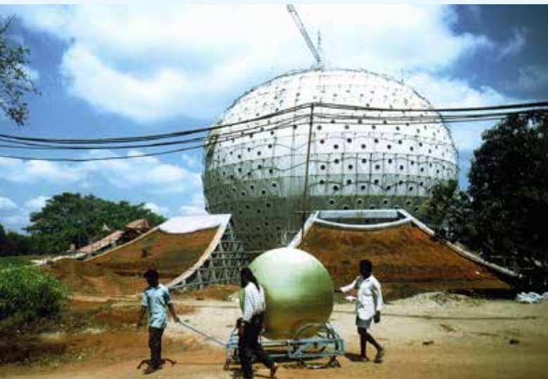
By 1996, the spherical space frame had been closed with prefabricated ferrocement panels. The first trials of mounting the golden discs on the outer shell began.
