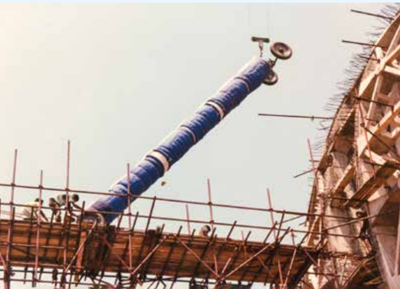
The twelve columns, each 9 meters long and bundled in protecting blankets, were lifted by crane into the Chamber and then hoisted upright in early August 1991.
