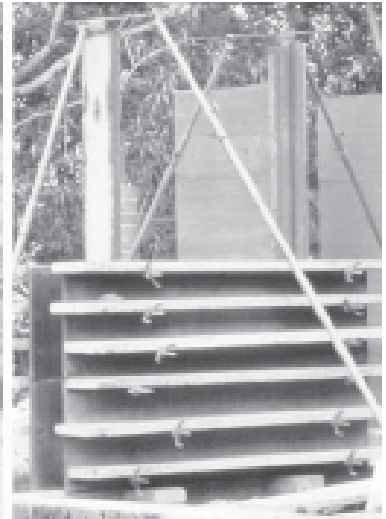
Rammed earth forms
