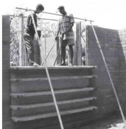
Stabilised rammed earth walls
