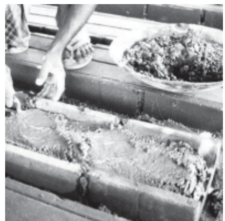
Composite lintels and beams
