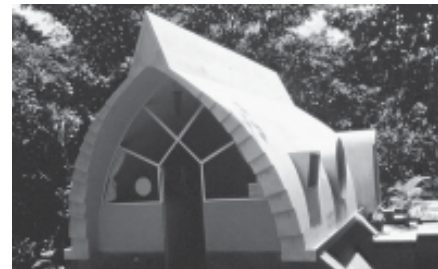
House at the Auroville Earth Institute
