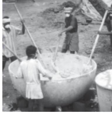
Stabilised earth waterproofing
