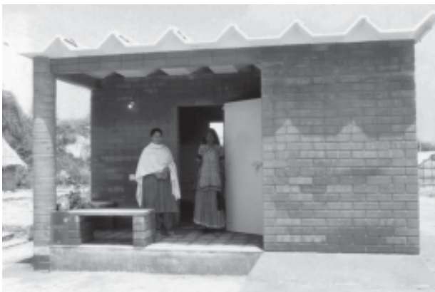
Improved AUM House - Khavda, Gujarat Built in 62 hours by an 20 man team
