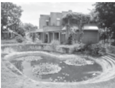
Biological wastewater treatment
