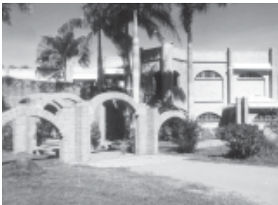
22 Domes of the Visitor's Centre
