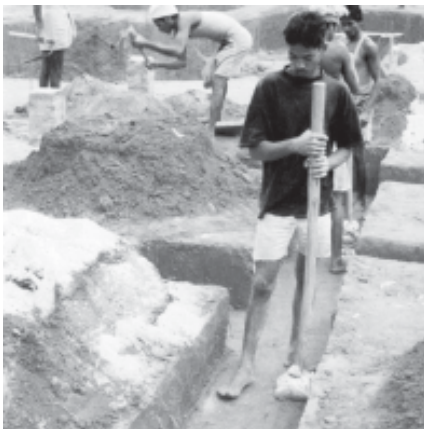
Stabilised rammed earth foundations
