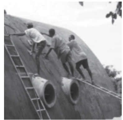
Stabilised earth waterproofing
