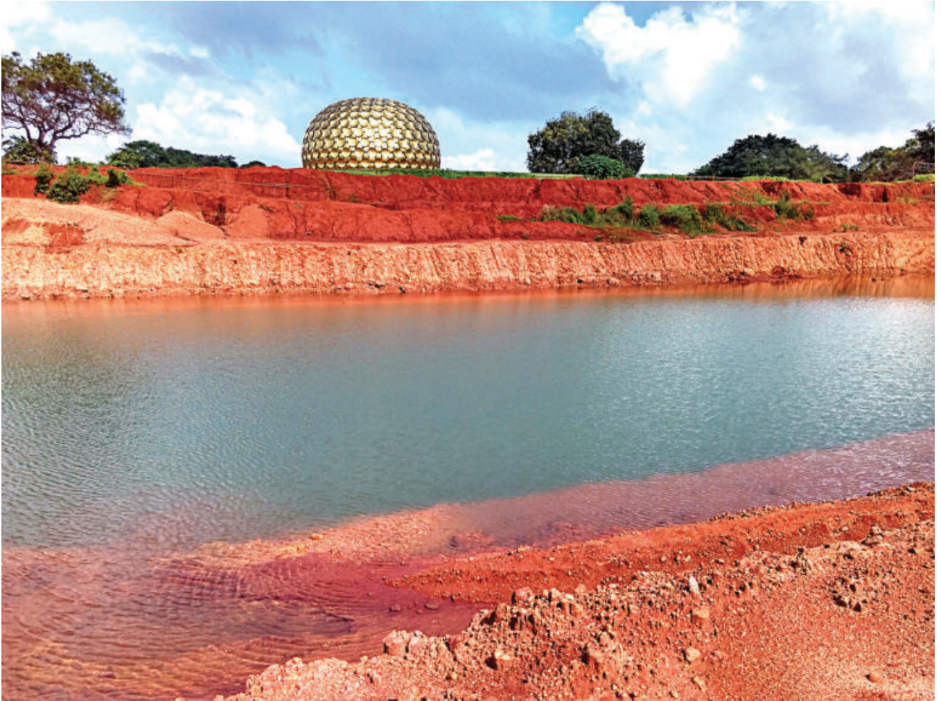
Clear ground water, over two meters deep, stands in the Lake excavation after the copious monsoon rains.
