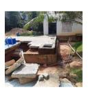
cumference of the pool in order to access and replace the old plumbing. The pump room will need to be modified and extended in order to easily access the new connections to the whole recirculating system. There are also other repairs
