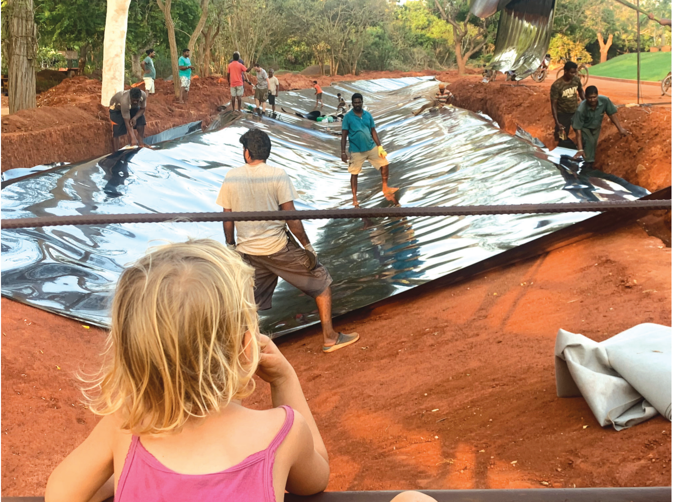
A young spectator watches from a temporary construction bridge as the water proofing liner is laid in the Open Water Channel which encircles the Matrimandir gardens.
