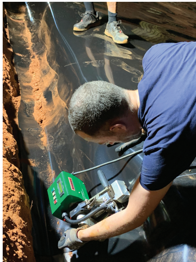
A self-propelled heat welding machine produced a double weld at the liner joints.
