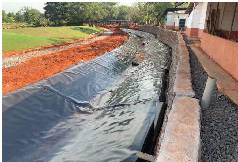
The V shaped channel was covered with a waterproofing layer.
