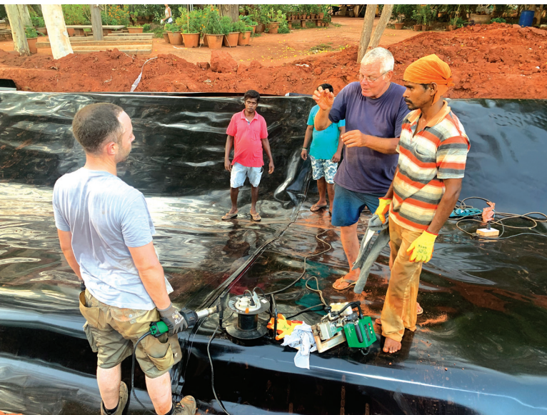
The joint welding team discusses the job.
