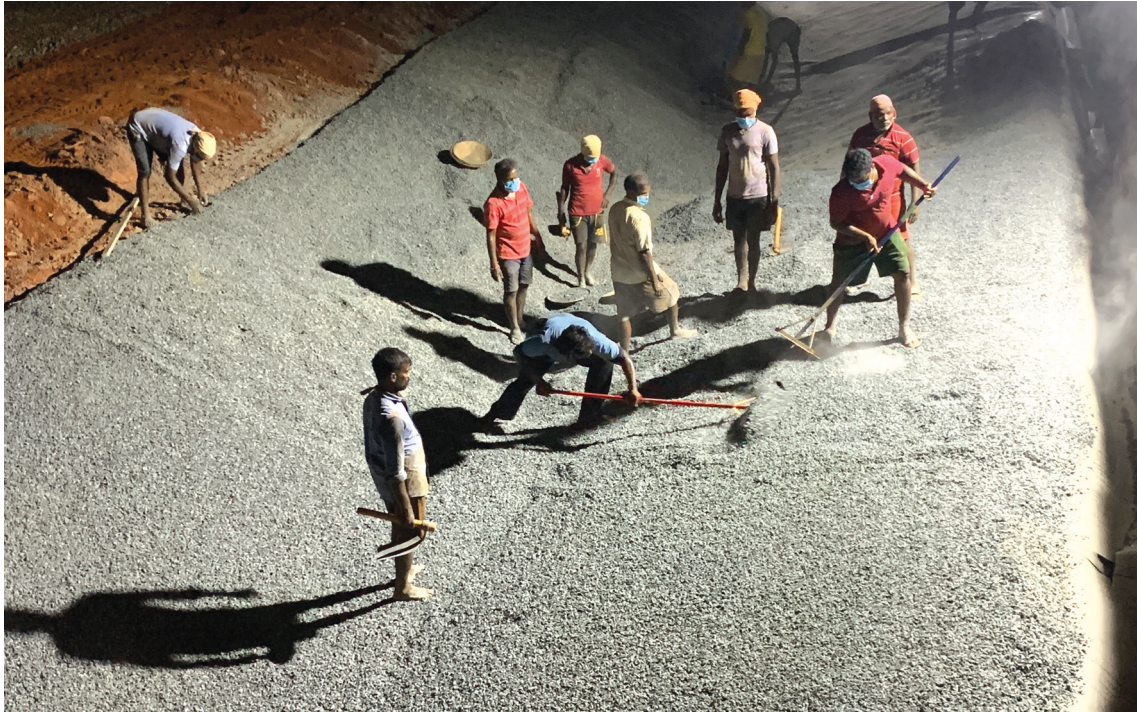
As a final step in the process, the HDPE line is covered with a 20 cm layer of granite chips to protect it from chances of puncturing and from the effects of UV radiation.
