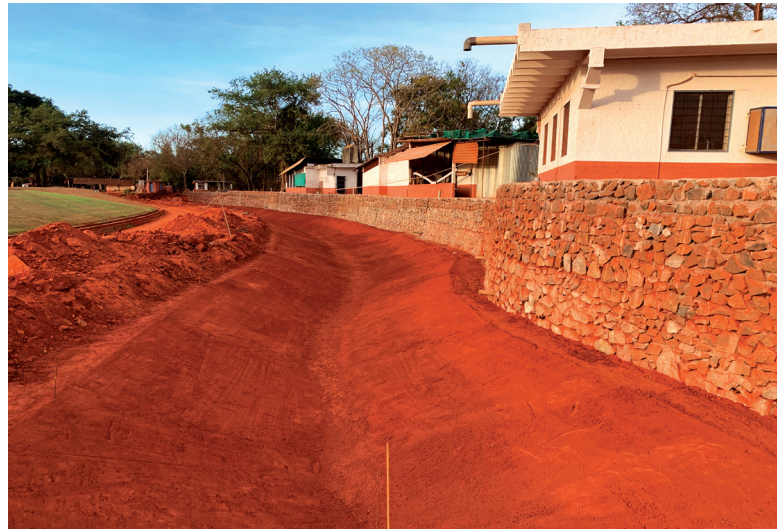
The V shaped water channel follows the newly built granite stone wall close to the Matrimandir workshops.
