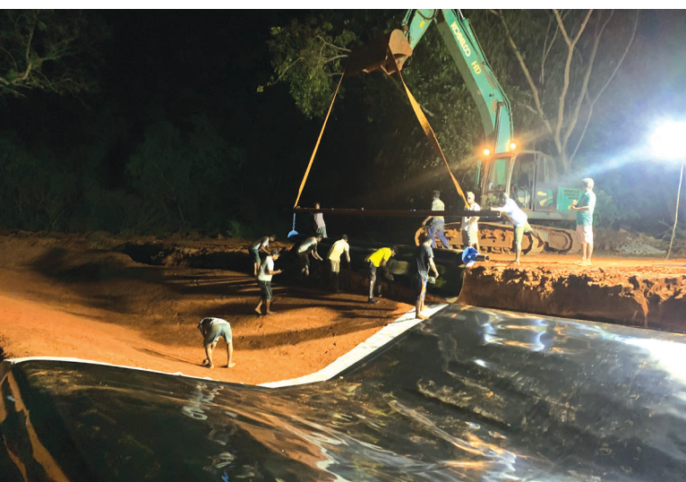
The laying of the liner took place at night, taking advantage of the cooler air to get the highest quality of welding on the joints.
